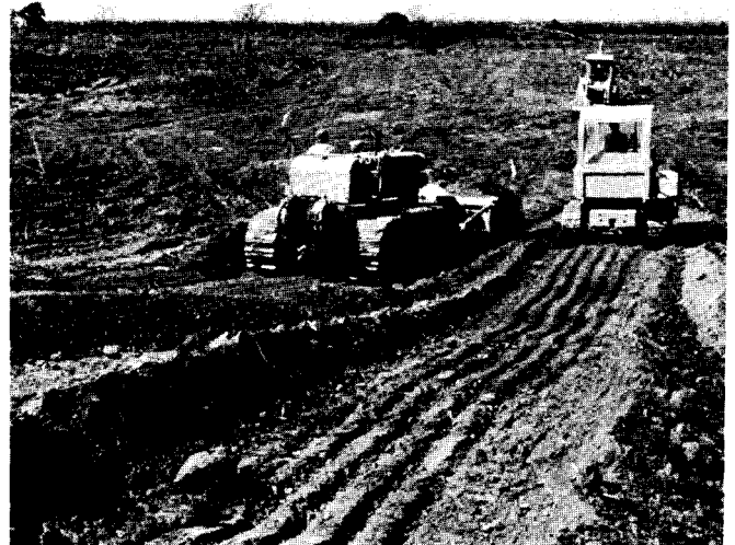
Figure 31. A pond in early stages of construction.
