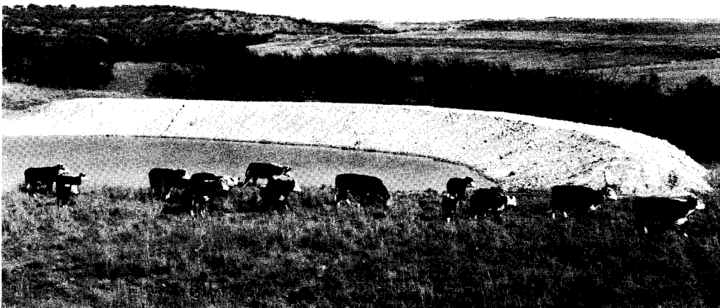
Figure 37. When vegetated, waste material on the windward side of a pond serves as a snow fence and a wind-break.
