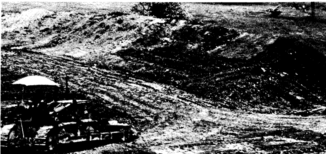
Figure 32. Sod and topsoil are stockpiled for later use.
