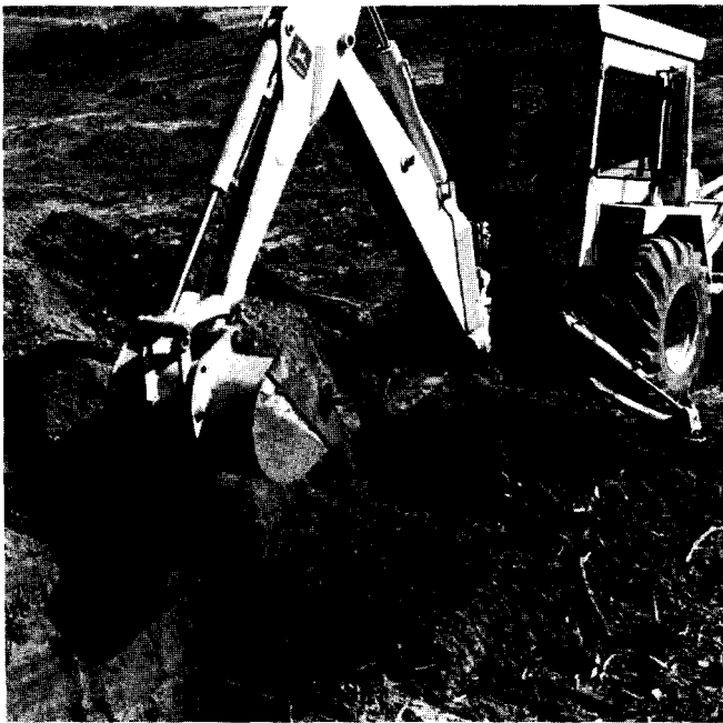
Figure 25. Cutting a core trench on the centerline of a dam.
