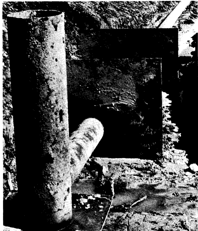
Figure 20. A drop-inlet trickle tube with antiseep collar.
