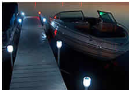
Residential dock w/solar Lighting
