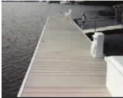
PVC Decking, power pedestal, dock box
