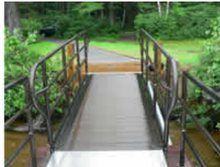
ADA style ramp w/anodized aluminum deck
