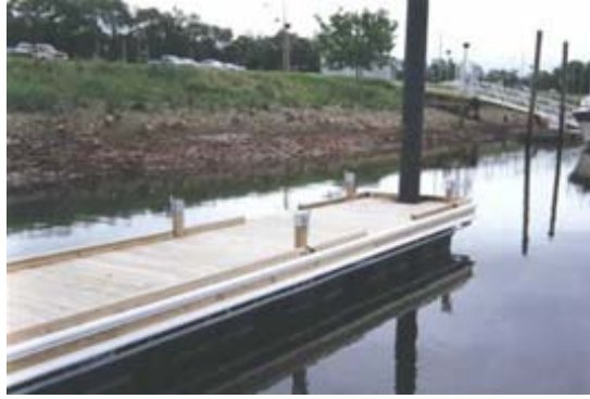
Steel piling support for end of ADA finger (w/deck rail)
