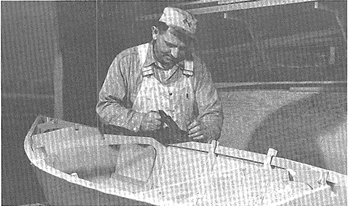
Fig. 4. Cut and screw on the gunwale fillers and cockpit corner knees, as shown on plans, then glue and screw these in place. Cut deck stringers and fasten them, then bevel them and edges of gunwale strips and frames to decking.
