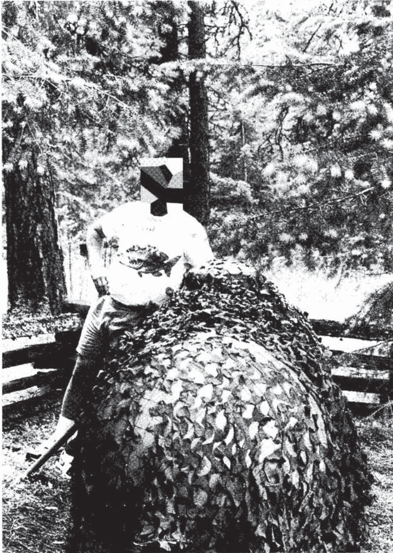
This retreator relies on his 1,000-gallon propane tank as one energy source. These tanks can also be coated with roofing compound and buried out of sight.
