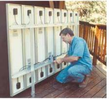
Take into account the location of the module junction box when installing modules to minimize interconnect wiring.
