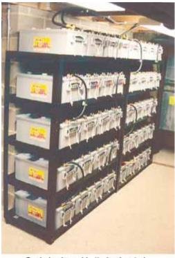
Sealed solar gel batteries located in an open basement rack
