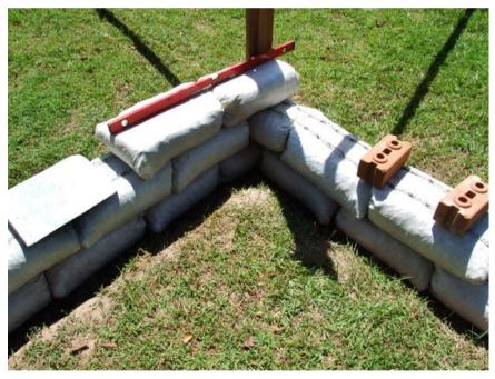
7. Repeat the process using earth-filled bags, but with a few minor changes: turn bags inside out to avoid protruding corners; use lightly moistened soil; tamp the contents slightly after each bucket load is added; pre-tamp each bag after it is aligned in position. This last step lengthens each bag to ensure good overlap.
