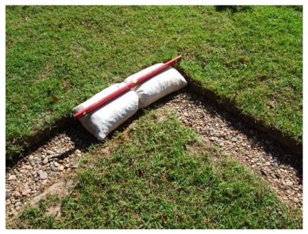
4. Lower courses: place gravel-filled bags (double bagged) working from the corners and openings to the center. It helps to tilt the first two bags against each other. Align bags to stringline; tamp the bags solid and level after the course is complete, working from the center of the bags outward. Always put tops of bags (the ends you've sewn closed) butted against other bags (never facing outward on corners or ends). Maintain a running bond as in masonry.
