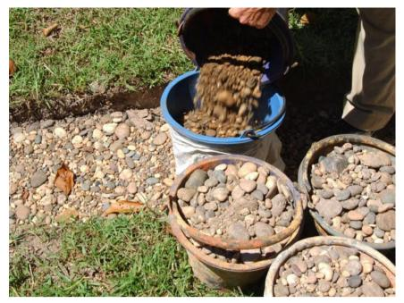
2. Fill the bags: use 2-gallon cement buckets to measure the fill material. Use the same number of buckets for each bag. Fill bags approximately 90% full, leaving just enough to sew the bags closed. This technique ensures a.) each bag is filled to capacity to save bags, and b.) each bag is the same size, which helps keep walls level. Bag stands are not needed.
