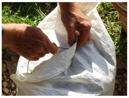
3. Sew or stitch the bags closed: fold the bag end over; use 15 gauge wire about 9" long with one end cut at a sharp angle; make one stitch on one side and bend the end over; make a stitch in the center and pull the corner over; make a stitch in the other corner and pull the corner over; poke the remaining wire into the earthbag. This technique facilitates handling, prevents spills and enables bags to be filled to capacity.
